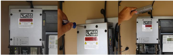
1. Remove to top two screws, and top cover plate. (as seen above).
